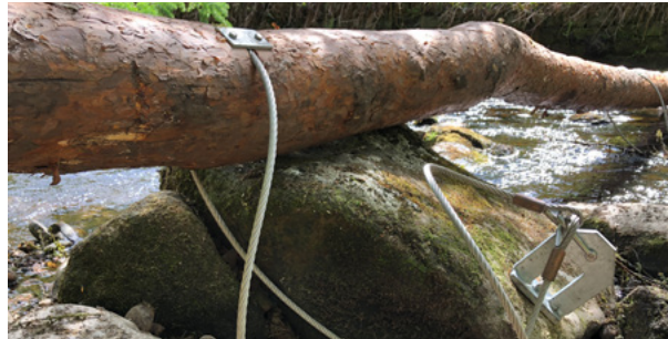
A log secured to the river bed to attenuate flow, Upper Calderdale (© National Trust Images)
