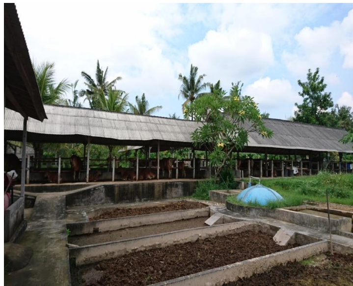
Figure 2. Cattle waste digester for processing cattle waste and yield biogas energy. The slurry resulting from digestion is processed for high quality fertilizer
